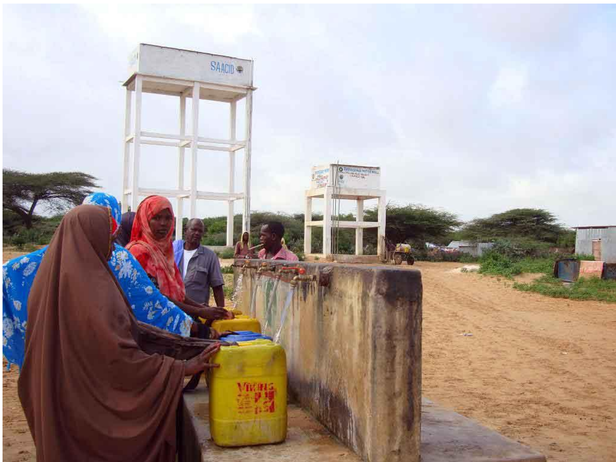
Water point with water tanks in the background
