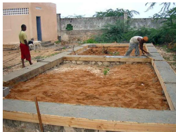
New schoolrooms being built in Deynile District
